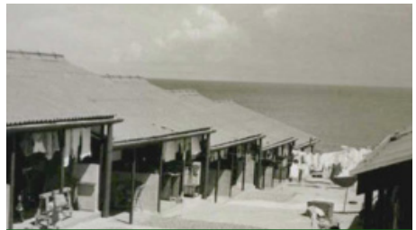
40 Houses and 20 Houses in 1951. The Buildings were removed following the 1988 Cyclone.
